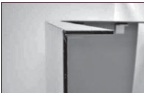
Cope at Edge of Panel
