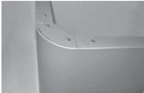
Corner Panel with Gusset & Filler Plate
