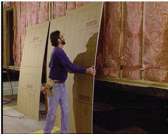
Preparing to install Backer Board.
