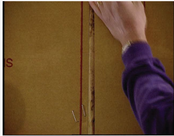
Moving Backer Board sheet into position. A gap may occur but is not required to positioning sheets across the next 4' section of wall.
